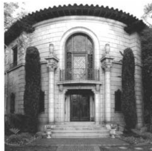
Petitfils-Boos Residence— A high-design property that will use its Mills Act savings to help support a significant rehabilitation
